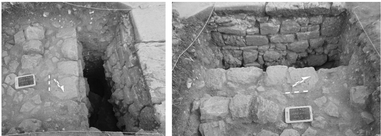
Fig. 7. The stylobate foundation exposed in Sond.2c.
