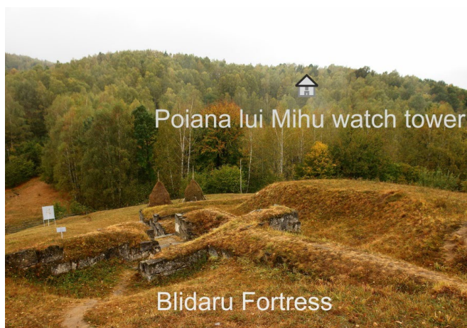
Figure 2. Position of the watch tower seen from inside of Blidaru Fortress.
