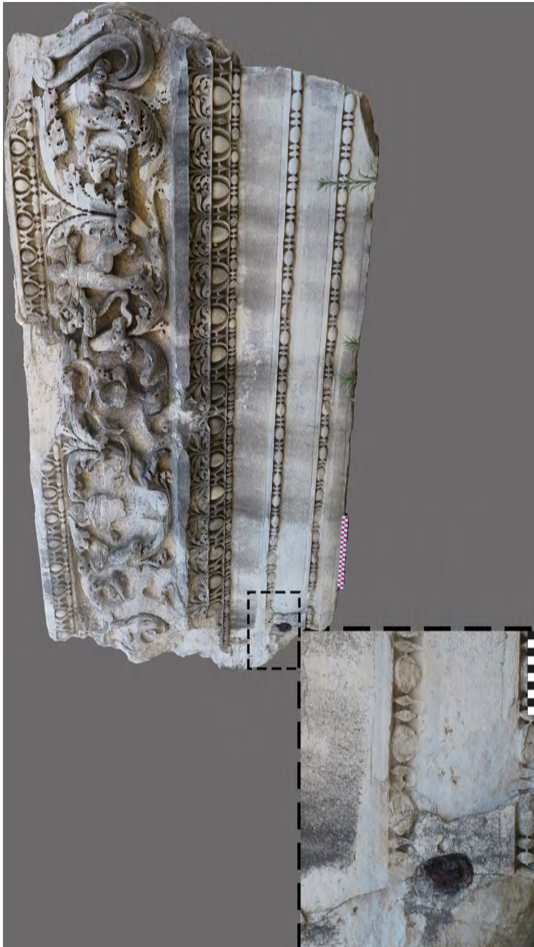
Fig. 3b. Ancient repairs on the structural elements of the Pergé theater.
