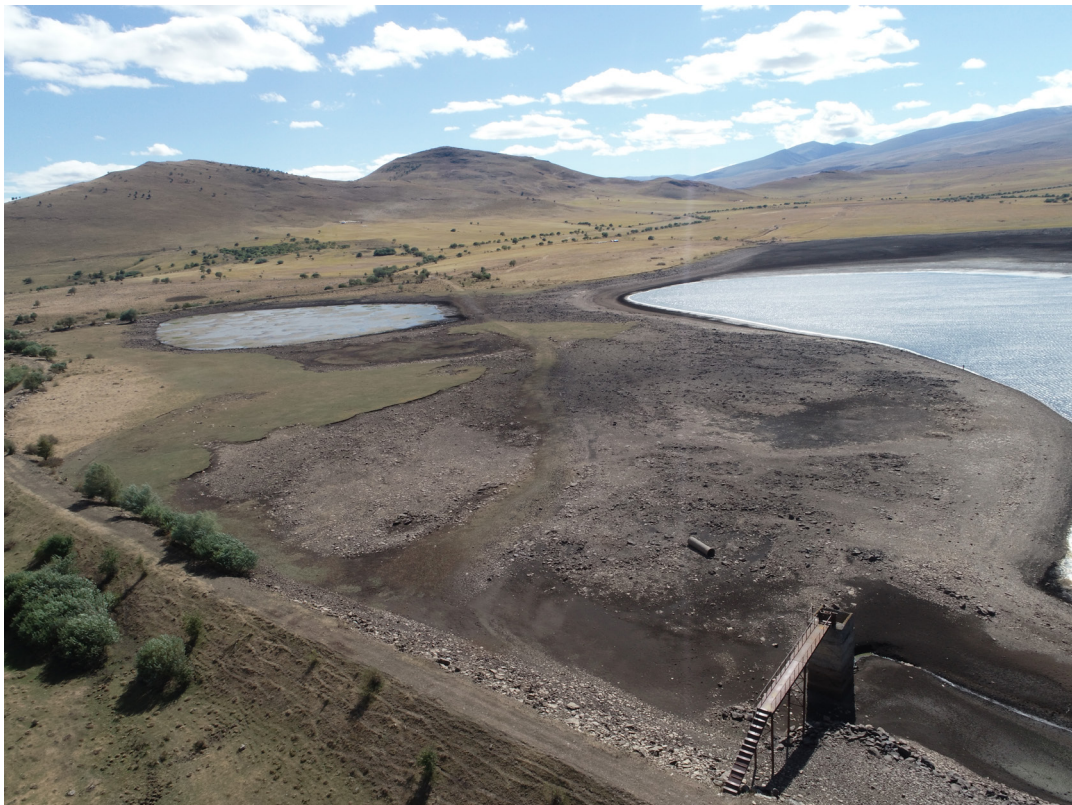
Fig. 4. Aerial photos of Bashplemi Lake shore.
